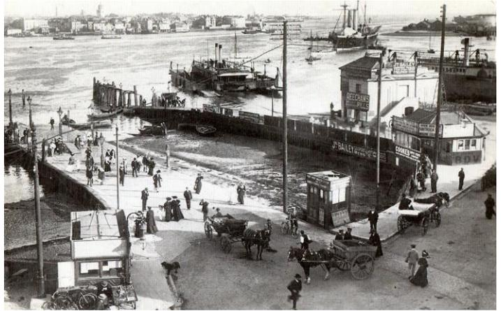
This ferry was steam-driven. Fixed chains across the harbour were pulled in and let out through the ship's engine, thus moving the vessel across the water. They were pulled over rollers and passed under the ship before falling back to the harbour bed. There were to be four ferries in all, spanning 1842 to 1959, the first two, *Albert* and *Victoria*, being replaced by *Duchess of York* and *Alexandra* – of which I have several memories...
